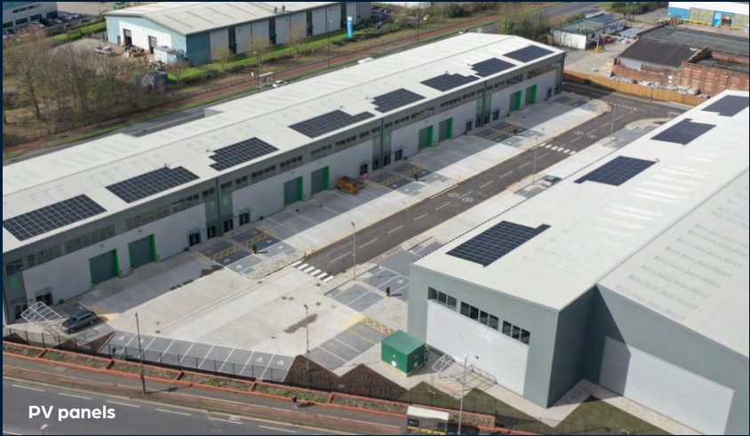
Warehouse roof lights
