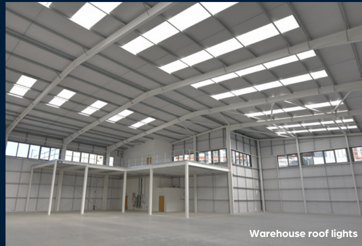
15% warehouse roof lights increasing natural lighting
